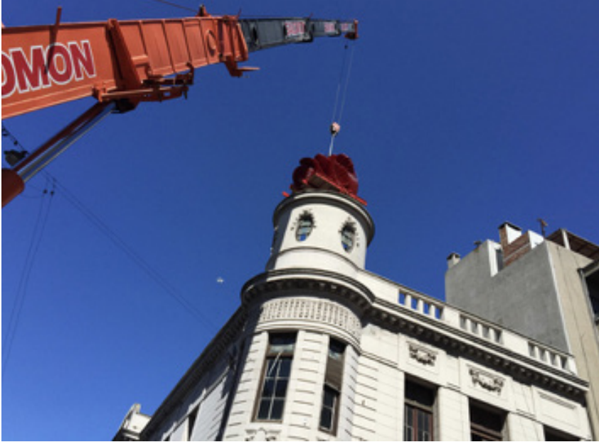
Figure 2 Installing the dome. Ph. Fernando García Amen, 2015.
